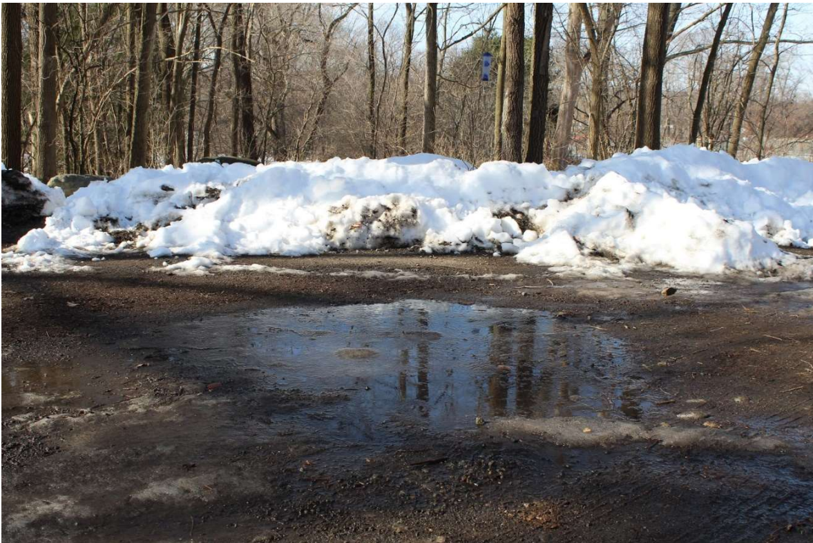
Figure 2.2. Lack of drainage due to erosion and potholing.
