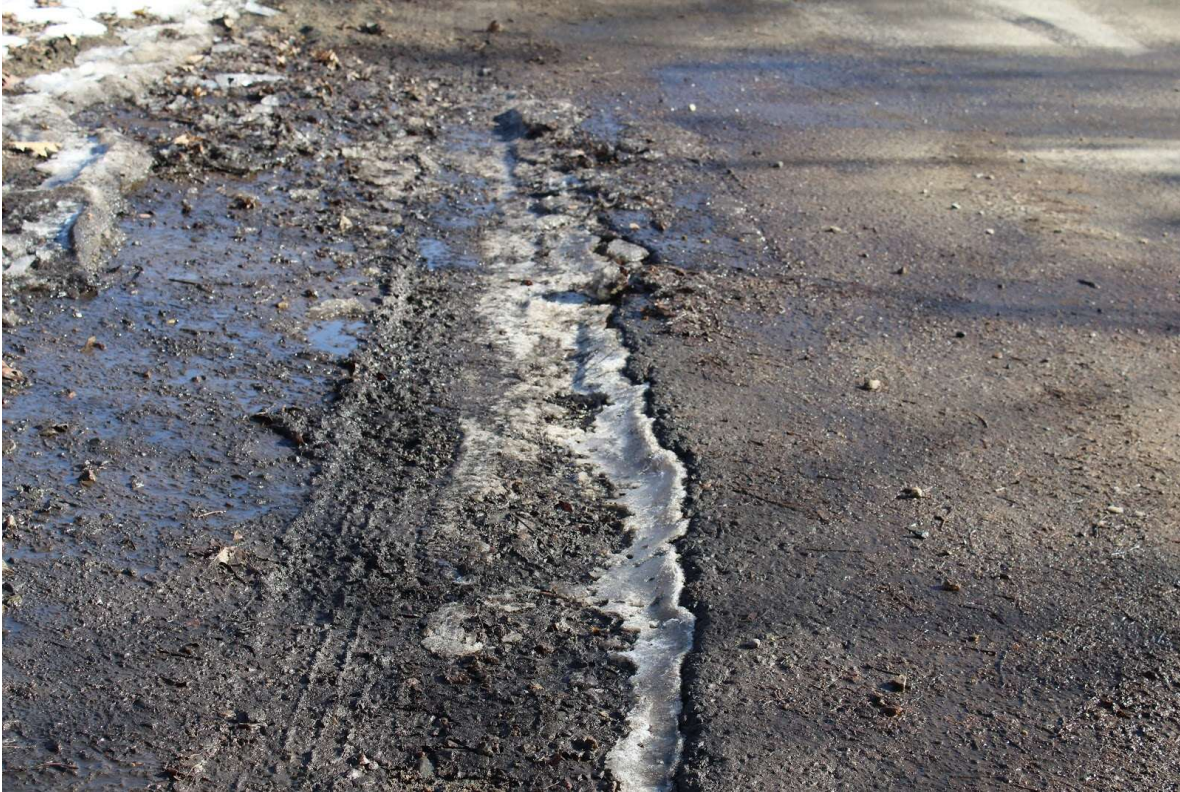
Figure 2.5. Inconsistent paving and erosion.
