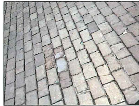
5. Damaged, cracked and broken Slate
