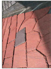
8. Damaged Slate & Mismatched Color
