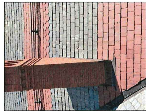
6. Typical Damaged Slate
