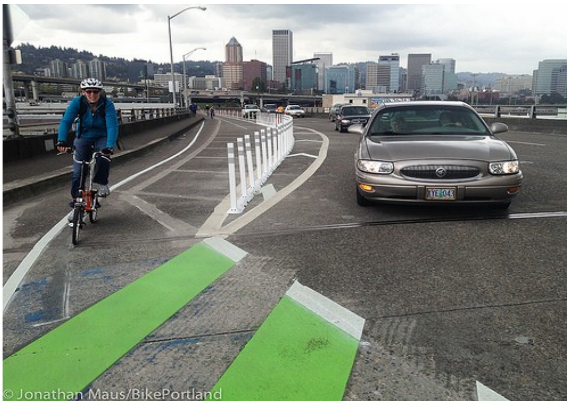
Illustration 2: Bollards placed between travel lane and bicycle lane to provide increased protection in bicycle lanes. Bollards would be designed for easy removal in winter to allow snowplowing.
